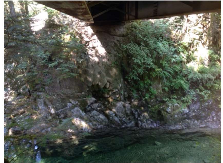
Right Bank Abutment when facing downstream
