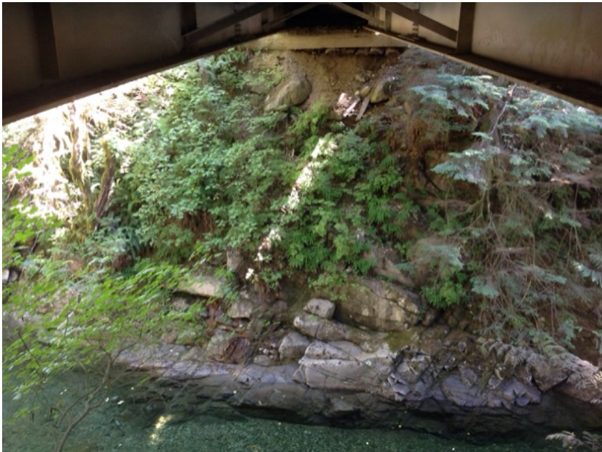
Left Bank Abutment when facing downstream
